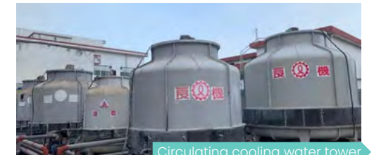
Circulating cooling water tower
